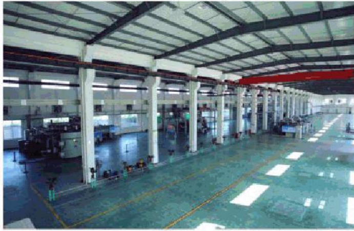
烧结车间 Sintering Workshop
